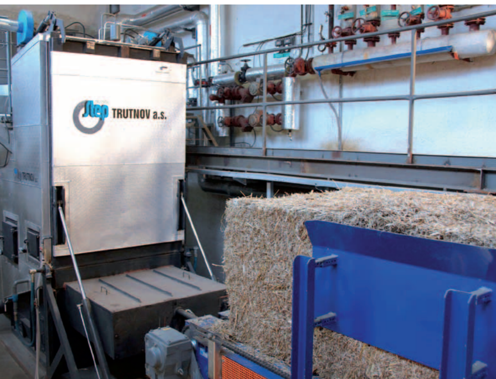
1/ An example of reference boiler plants for burning whole bales of straw, hay, flax, pressed paper boxes, etc. can be found in Častrov u Pelhřimova. In addition to the Gold Product Award of Česká stavební akademie [Czech Construction Academy], Step TRUTNOV is the holder of Gold Stevie® Award 2012 , Bronze Stevie® Award 2013 and others.
